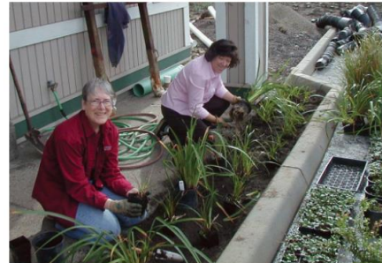
Bioretention during installation
