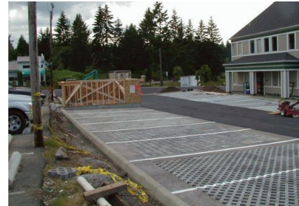
Permeable pavement installation
