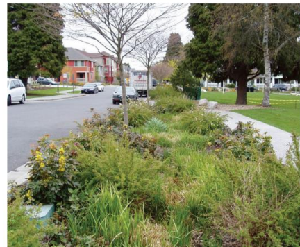
Established bioretention facility
